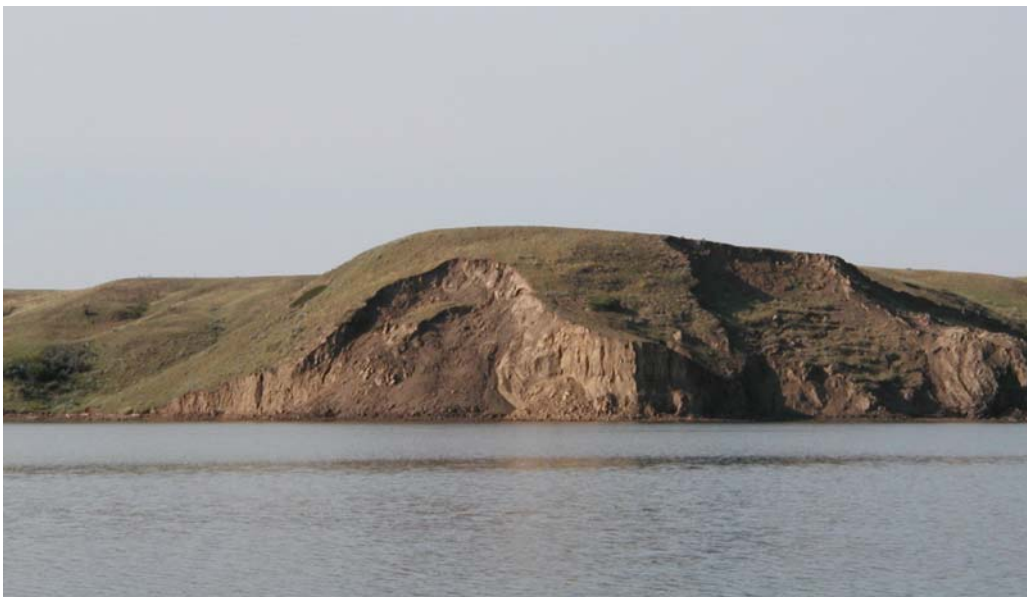
Figure 9.3. Large areas of erosion above the reservoir maximum water surface (photo by S. Nuanes).
